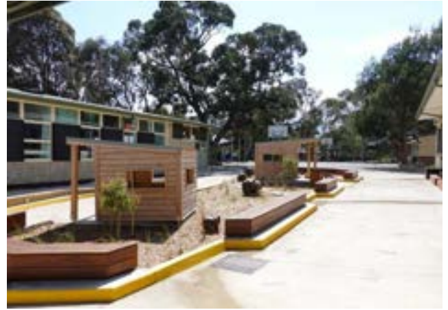
A recently completed play area with cubbies, wooden sculptures of Australian animals and seating may appear stark, but a couple of eucalypts have been planted and in time will provide welcome shade. Resilient lomandras have also been used to soften the space.
