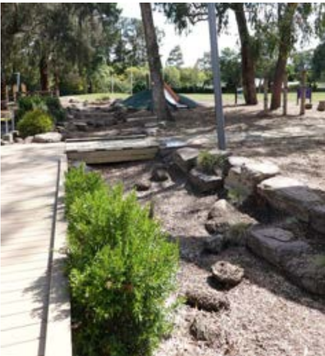
A dry river bed is both aesthetically pleasing and takes care of stormwater.
